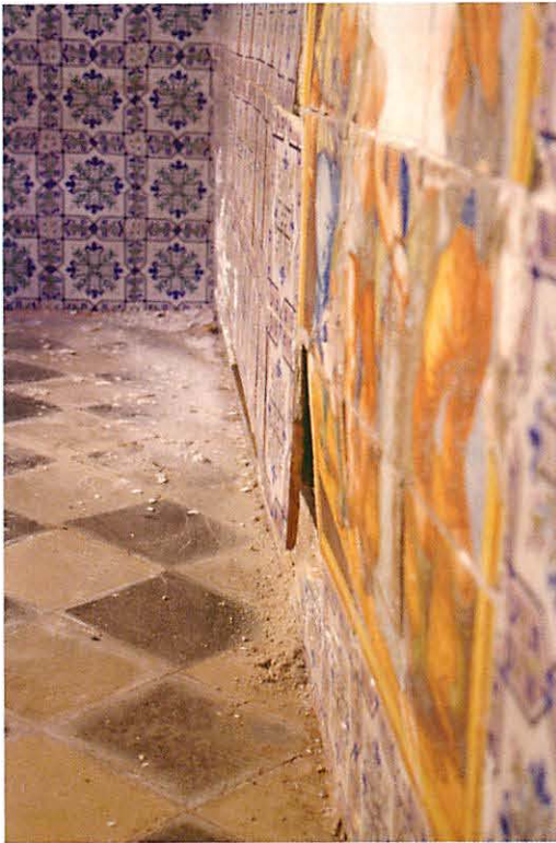
Fig. 6: Bombaments i desprendiments
